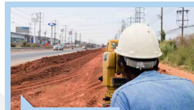
Adana - Kozan Road Work
